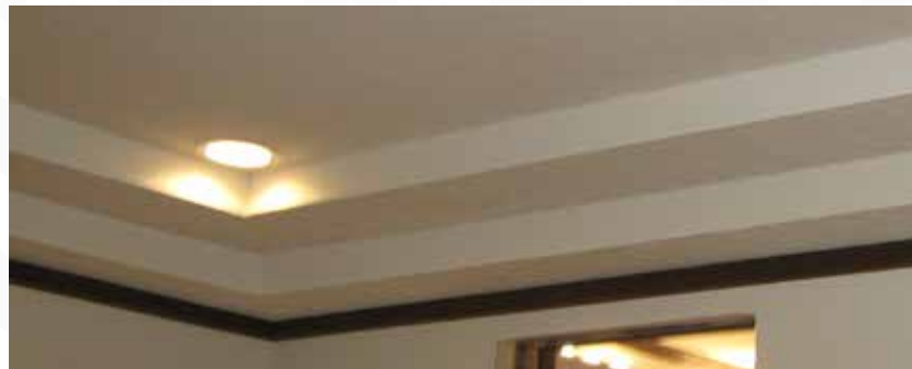
2 Tier Soffit with Can Lights
