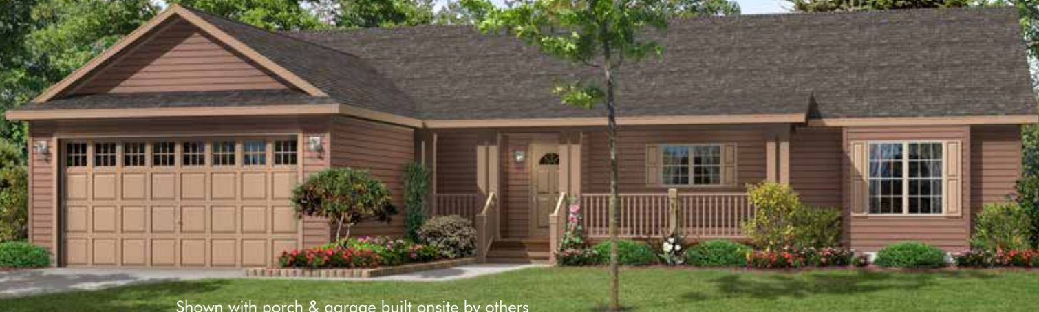
Shown with porch & garage built onsite by others
